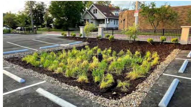
The La Salle parking lot retrofit included bioretention cells and underground chambers that drain 0.55 acres and helps capture 166,000 gallons of water a year.
