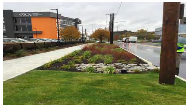
The LINK 59 project included bioretention cells that drain an acre of land and help capture 582,459 gallons of stormwater a year.
