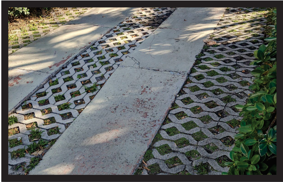
Figure 1154-01: Graphic showing paving materials for a residential driveway. In this example, the main drive treads were paved in concrete, whereas the adjacent areas were paved using concrete pavers that allow for some stormwater infiltration—a “stormwater-wise” technology.
